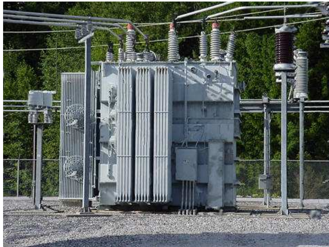
Figure 9.20: Substation transformer.
